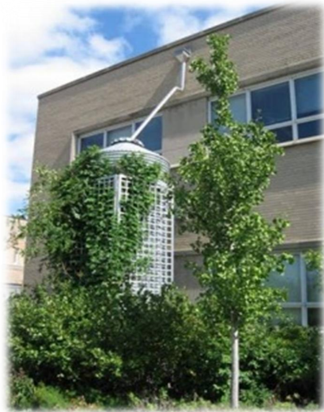
Cistern at the Chicago Center for Green Technology (Source: Abby Hall, U.S. EPA) Source: https://www.werf.org/liveablecommunities/toolbox/rainbarrel.htm
