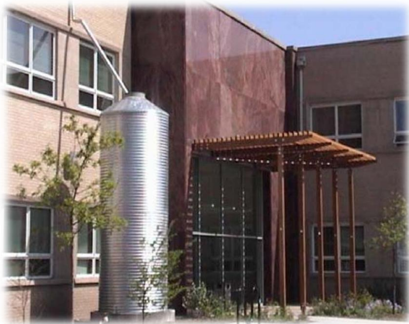
A cistern at the Chicago Department of Environment Source: werf.org
